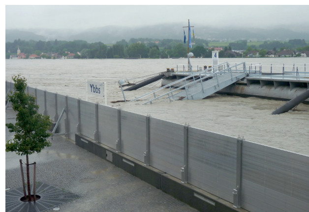
Ybbs power station stage - 4th June 2013
